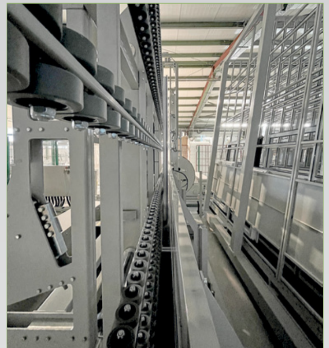
The elements are temporarily stored in the distribution buffer system.
